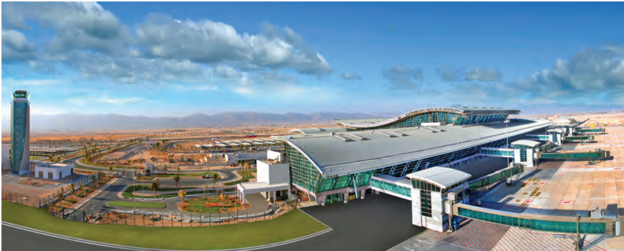
Standby Power at Salalah Airport.
