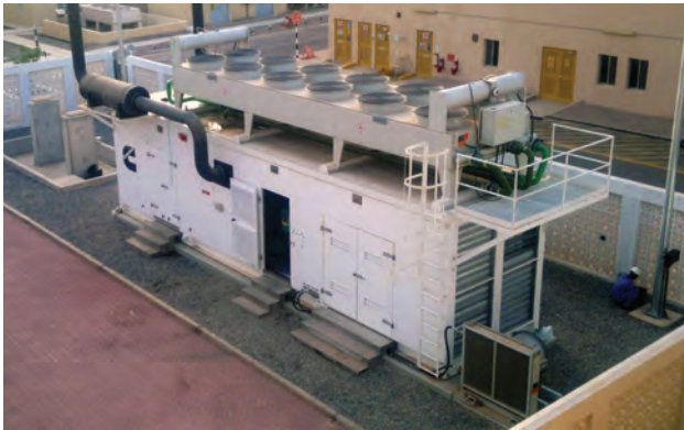
Backup generator with Fire detection and suppression system thermostatic controlled cooling system and complex utility changeover control with bump less restoration at PDO Mina Al Fahal.
