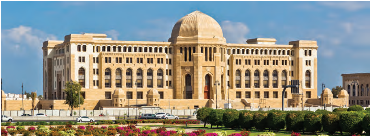
Standby Power at Supreme Court building
